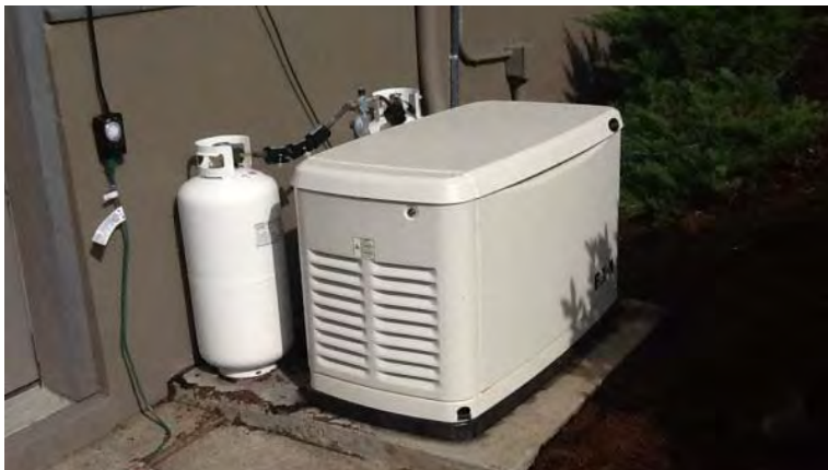
Figure 6 Propane-Powered Generator
